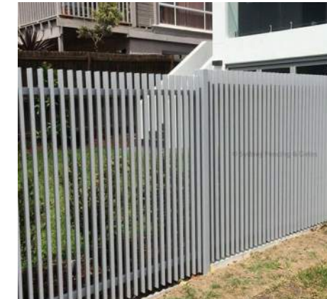
ALUMINIUM SLAT FENCE FINISH: COLORBOND SURFMIST LOCATION: PERIMETER
